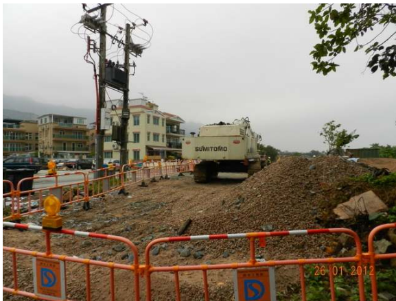
Photo 1 – Temporary hoardings have been erected around the active works area.
