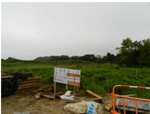
Photo 3 – Wetland rehabilitation area was observed adjacent to the active works area.
