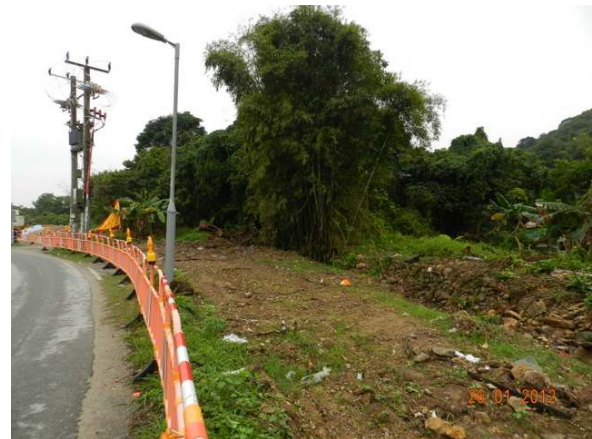
Photo 2 - Temporary hoardings have been erected along Tung Tsz Road.
