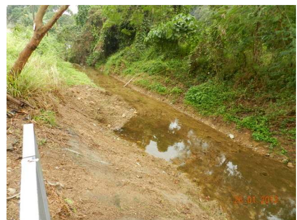
Photo 6 – Stockpiled soil was still observed at the bank of the Wai Ha.
