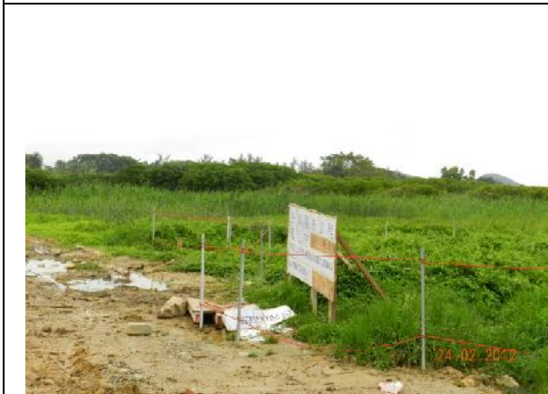
Photo 3 – Wetland rehabilitation area was observed adjacent to the active works area.
