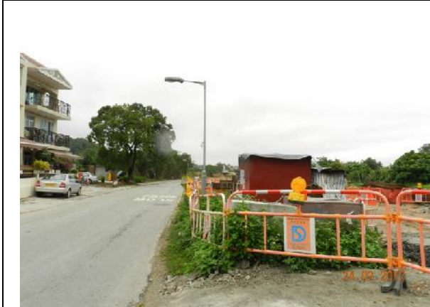
Photo 1 – Temporary hoardings have been erected around the active works area.
