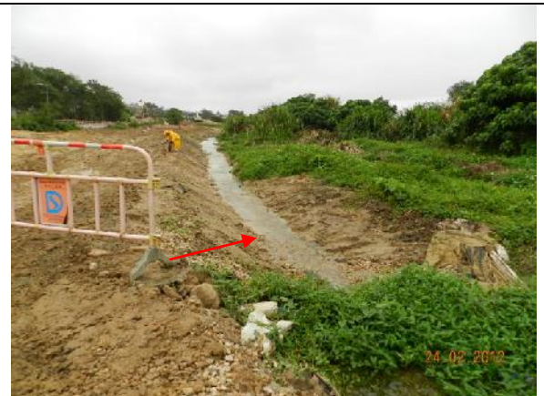
Photo 4 – Sedimentation tank for water drained from the underground was removed.
