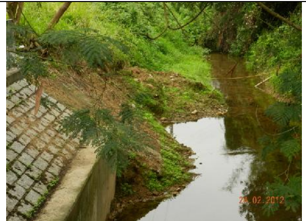
Photo 6 – Stockpiled soil was still observed at the bank of the Wai Ha.
