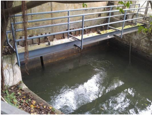
Photo 1. Wai Ha River at W2
