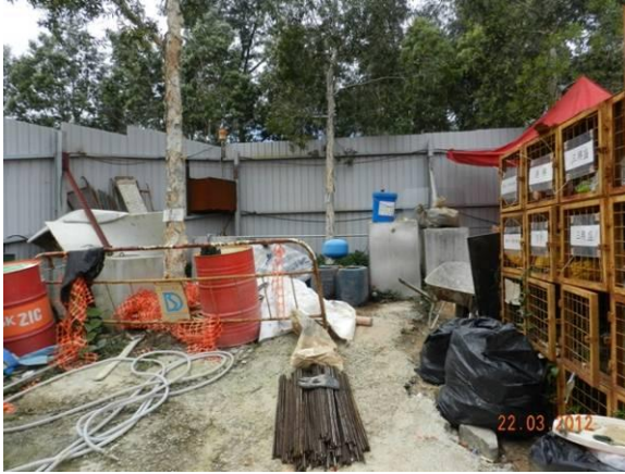
Photo 7 – Temporary stored construction materials were observed within the TPZs in Area A.
