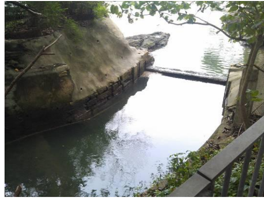
Photo 2. Wai Ha River at W2
