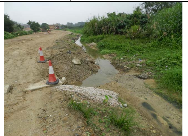
Photo 6 – A few sections of sedimentation beds with gravels was observed.
