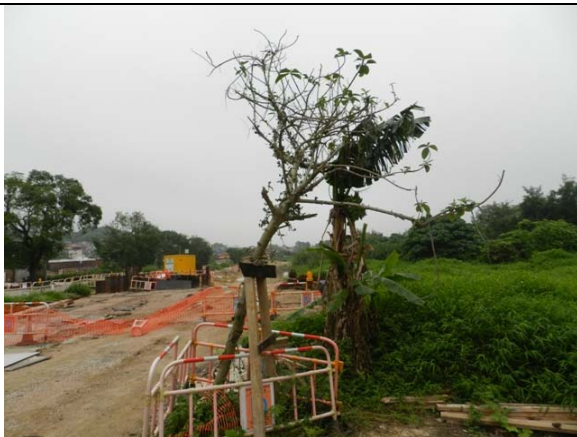
Photo 17 – The temporary site office near the leaning retained tree T190 ( Ficus hispida ) was found relocated to the southwest of the retained tree T196. The tree was still found being supported by a wooden stand.
