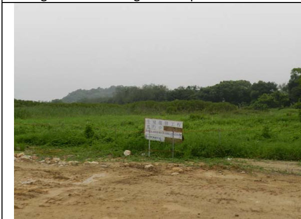
Photo 5 – Wetland rehabilitation area was observed adjacent to the active works area.
