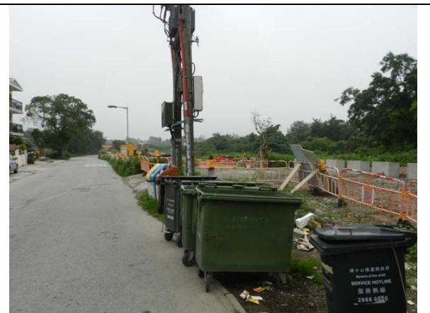
Photo 2 – Temporary hoardings have been erected around the active works area.
