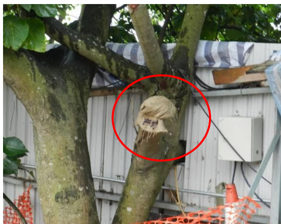
Photo 11 – The injured part of the retained tree E44 was found pruned and wrapped by burlap
