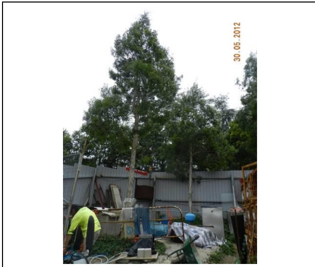
Photo 7 – Temporarily stored construction materials were still observed within the TPZs in Area A.
