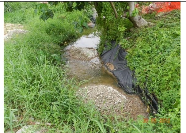
Photo 6 – The sedimentation beds and PVC liner were aligned from north to south near the retained tree T196 ( Macaranga tanarius var. tomentosa ).
