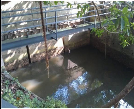
Photo 3. Wai Ha River at W2
