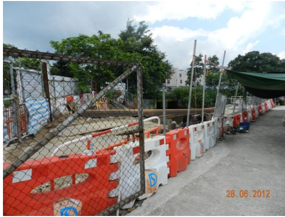
Photo 1 – A temporary hoarding was established to surround the works area at Wai Ha River estuary.
