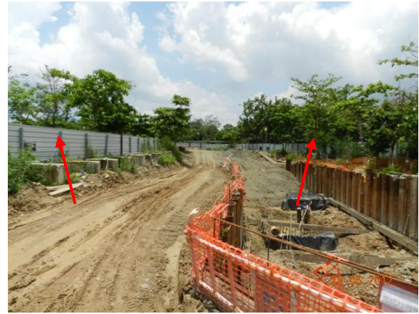
Photo 2 – A temporary hoarding was established to surround Area B within Tung Tsz Nursery.
