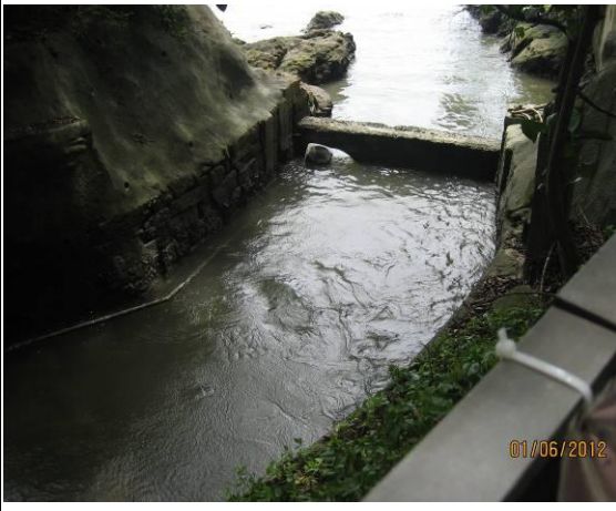
Photo 2. Wai Ha River at W2
