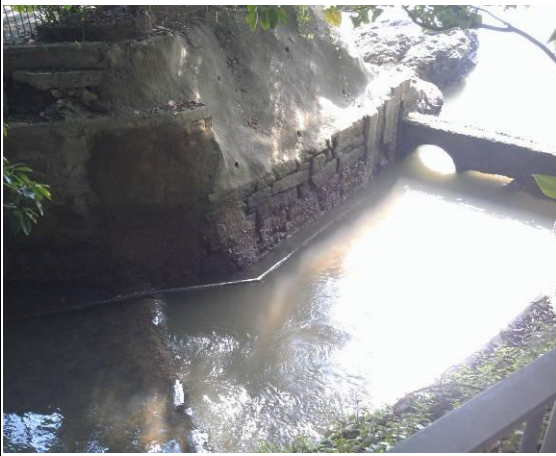
Photo 4. Wai Ha River at W2
