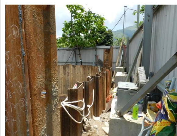
Photo 17 – Relocated trees were unable to be assessed closely due to the construction of the box culvert.
