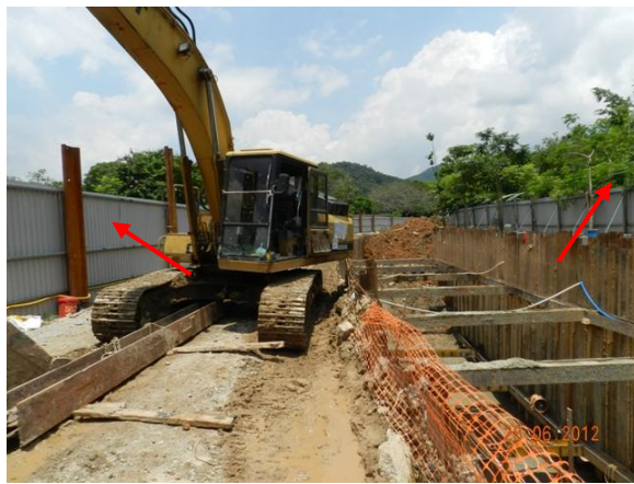
Photo 3 – A new section of temporary hoarding has been erected from southwest to eastern parts of the Tung Tsz Nursery.
