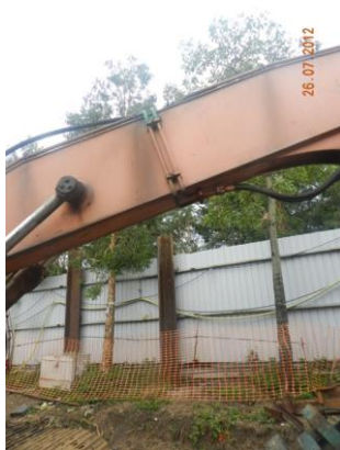
Photo 11 – Temporarily stored construction materials were no longer observed within the TPZs in Area A.
