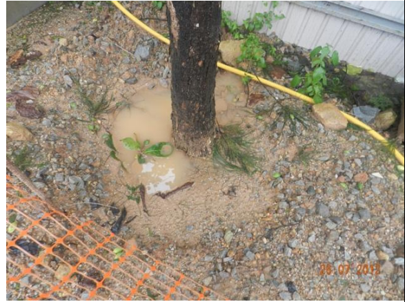
Photo 20 – Waterlogged area was observed at the base of U79.
