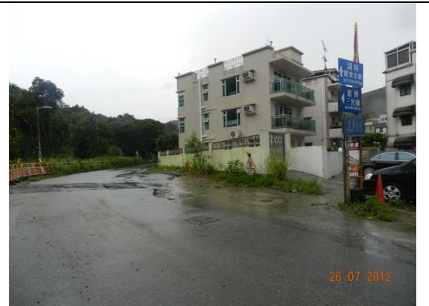
Photo 4 – Temporary fences were removed during the monitoring on 26 th July 2012 as the works in the area was finished.
