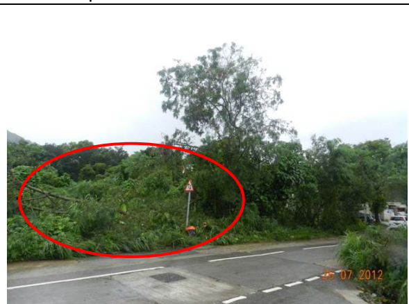
Photo 12 – Trees to be retained (T082-T084) were found fallen after the severe Typhoon 'Vicente'.
