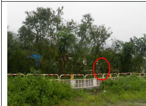
Photo 11 – Tree to be felled (T22) was found fallen after the severe Typhoon 'Vicente'.
