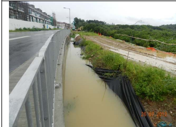
Photo 9 – The sedimentation beds and PVC liner were aligned from western to eastern parts along Tung Tsz Road and opposite to San Tau Kwok. The beds were overflowed by the rain.
