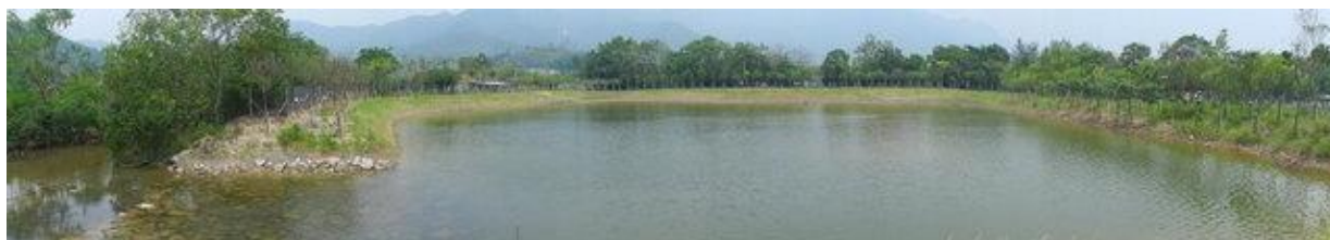
Photo 2. General view of the wetland as inspected on 21 st August 2012.
