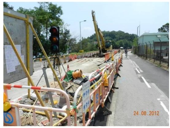
Photo 2 – Temporary hoardings have been established to active works area along Ting Kok Road.
