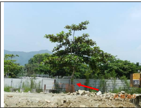
1.1.1 Photo 25 – The untagged tree next to U54 have been surrounded by the orange construction nets to prevent further damage to the tree trunk.
