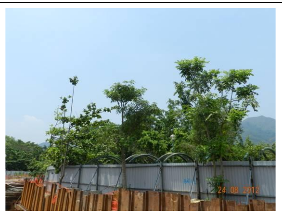
Photo 20 – General view of the relocated trees behind the sheet piles in Area B.
