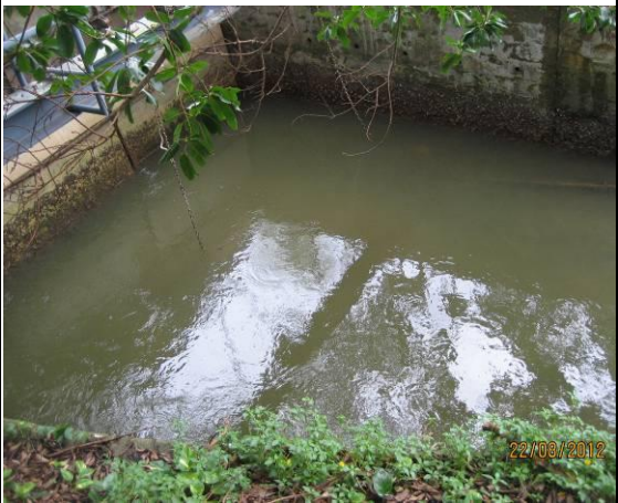
Photo6. Wai Ha River at W2
