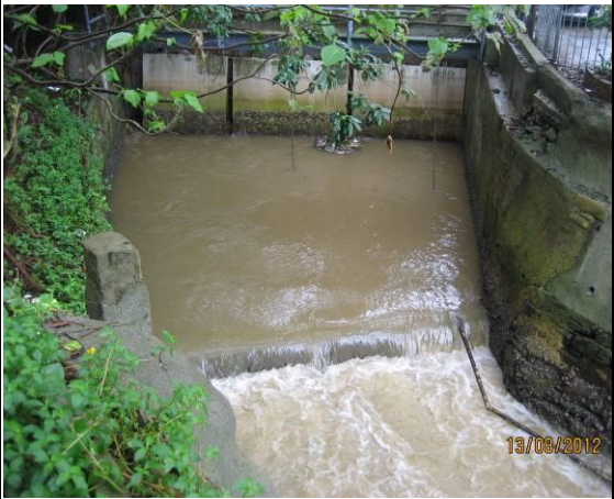
Photo 4. Wai Ha River at W2
