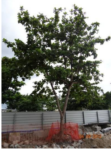
Photo 19 – The untagged tree at the south of U54 has been surrounded by the orange construction nets to prevent further damage to the tree trunk.
