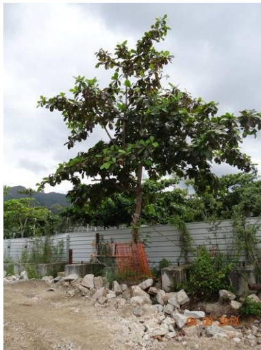
Photo 21 – The untagged tree at the north of U54 has been surrounded by the orange construction nets to prevent further damage to the tree trunk.
