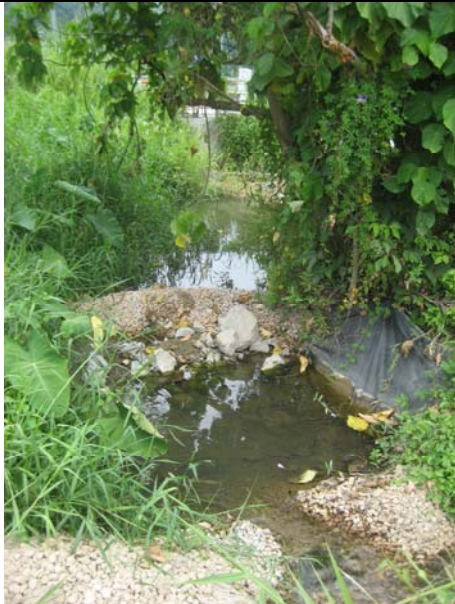
3. The rock bund in the de-silting channel has been repaired.
