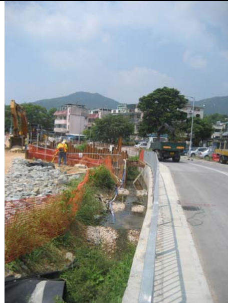
4. The de-silting channel was found to be cleaned.
