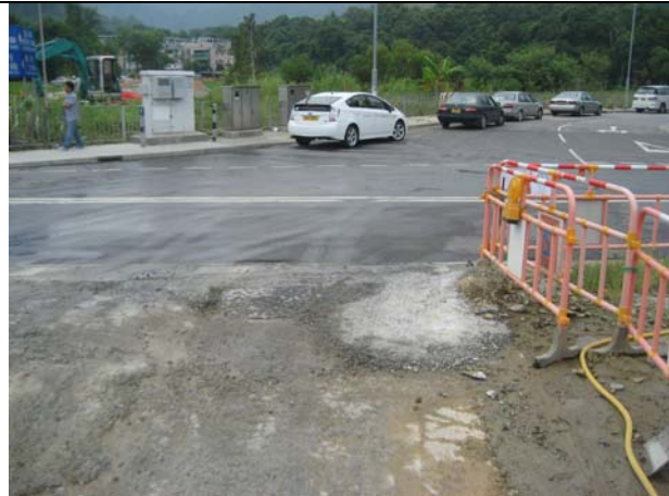
Observation 1. Regular watering spraying should be applied at the site exit/ entrance.
