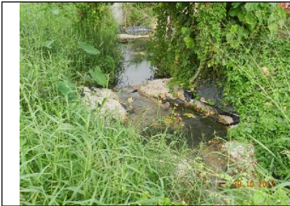
Photo 7 – The sedimentation beds and PVC liner were aligned from north to south near the retained tree T196 ( Macaranga tanarius var. tomentosa ) and no muddy water was discharged.
