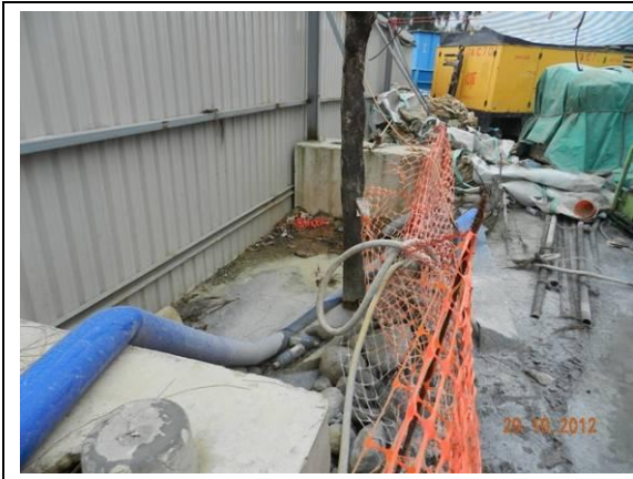
Photo 19 – The base of the tree U77 was waterlogged with used water from the construction work.
