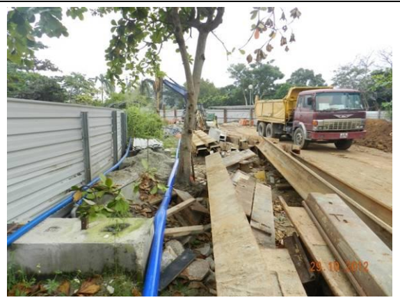
Photo 20 – Stockpiling of construction materials were observed immediately next to the trunk and damage was observed near the tree U54 and two existing trees with no tag next to U54
