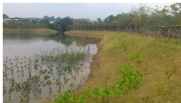
Photo 3. The ECA as inspected on 16 th October 2012.
