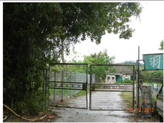
Photo 2 –The gate of the adjacent area near the previous main entrance of Area C has been reinstated to its original location.
