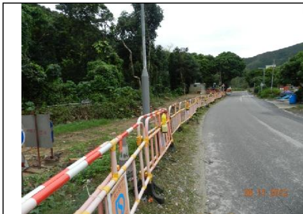
Photo 1 – Temporary hoardings have been erected around the active works area to the south of Wai Ha.
