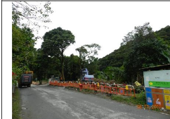
Photo 3 – New temporary hoardings have been erected along the west of Tung Tsz Road near the refuse collection point.
