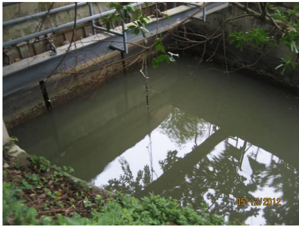
Photo 1. Wai Ha River at W2
