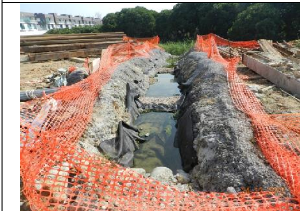
Photo 9 – The sedimentation beds with gravels and PVC liners was aligned from the area opposite to the Jade View Villa towards the marsh area at southeast.
