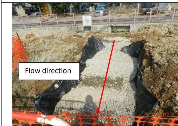
Photo 11 – The sedimentation beds with gravels and PVC liners was aligned from the area opposite to the eastern part of Jade View Villa towards the marsh area at southeast.
