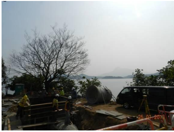
Photo 1 – Removal of site hoarding along the eastern boundary of Area A.
