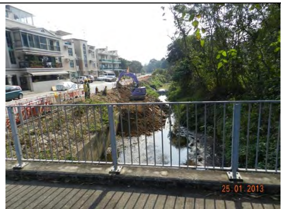
Photo 14 – Works have been commenced in Wai Ha River.
