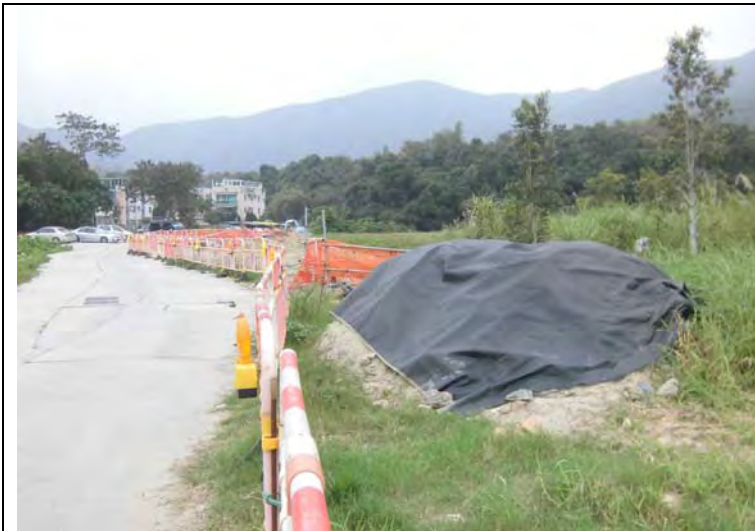
Photo 1: The sand stockpile has been covered with tarpaulin sheet.
