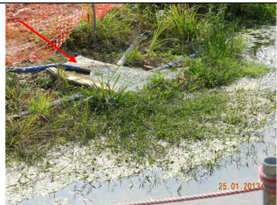
Photo 18 – Discharge of filtered water from the works area into the wetland rehabilitation area.
