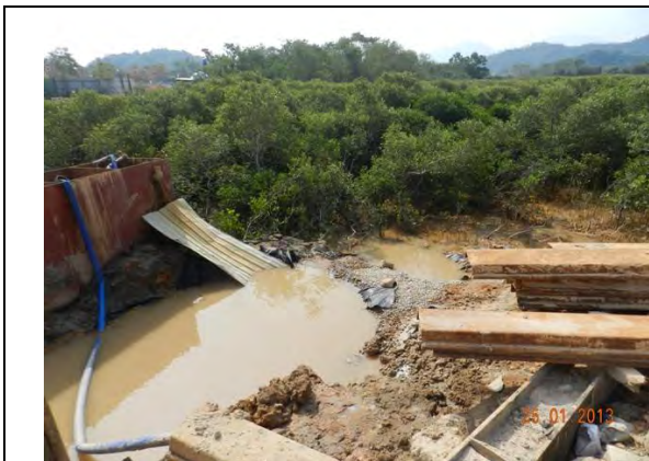
Photo 13 – The filtrate from the filtration tank was then run along a sedimentation bed and discharge into the vegetated area. The discharge was found muddy.
