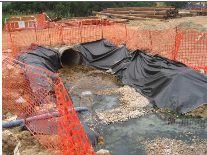
Photo 1: The general refuse inside the de-silting channel has been removed.
