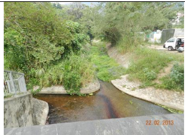
Photo 16 – No discharge of used water was observed at the upper section of Wai Ha River (i.e. to the north of Tung Tsz Shan Road).
