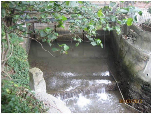
Photo 1. Wai Ha River at W2
