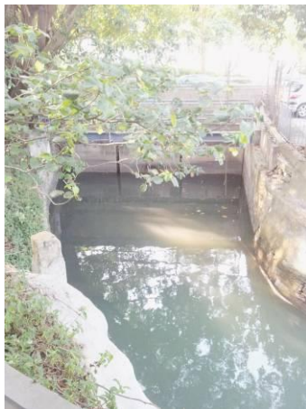
Photo5. Wai Ha River at W2
