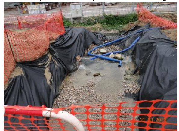
Photo 10 – The sedimentation beds with gravels and PVC liners were aligned from the area opposite to the eastern part of Jade View Villa towards the marsh area at southeast. The used water released to the sedimentation beds was generally clean.
