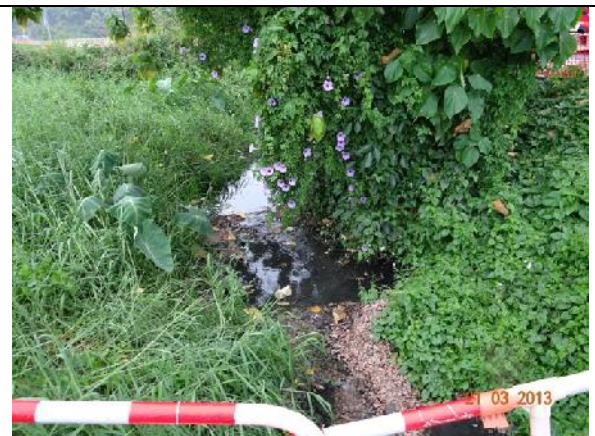
Photo 8 – The sedimentation beds and PVC liner were aligned from north to south near the retained tree T196 ( Macaranga tanarius var. tomentosa ) and no muddy water was discharged.
