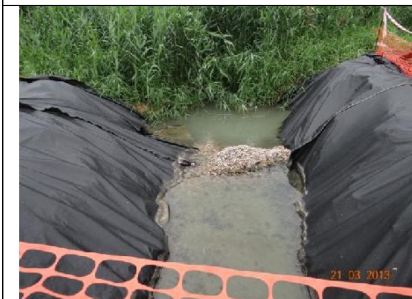
Photo 11 – The sedimentation beds with gravels and PVC liners was aligned from the area opposite to the eastern part of Jade View Villa towards the marsh area at southeast. The discharge was generally clean.
