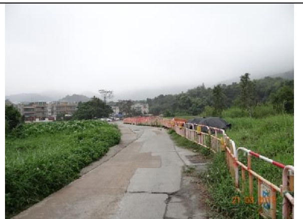
Photo 2 – Temporary hoardings have been erected around the active works area along the access road to Treasure Spot Garden II.
