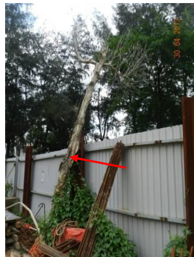
Photo 18 – Poor condition of the relocated tree T102 as observed within the Phase 2 works area of Area B.
