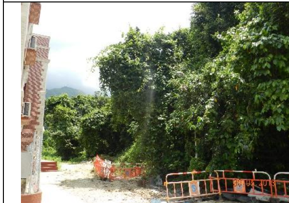
Photo 3 – Temporary hoardings have been erected on the path near Treasure Spot Garden II.
