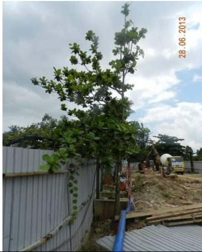
Photo 25 – Stockpiling of soil close to the trunk flare of A43 was still observed.
