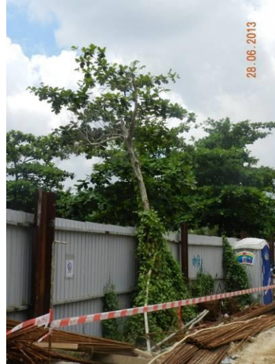
Photo 16 – Very poor condition of the relocated tree T102 as observed within the Phase 2 works area of Area B.
