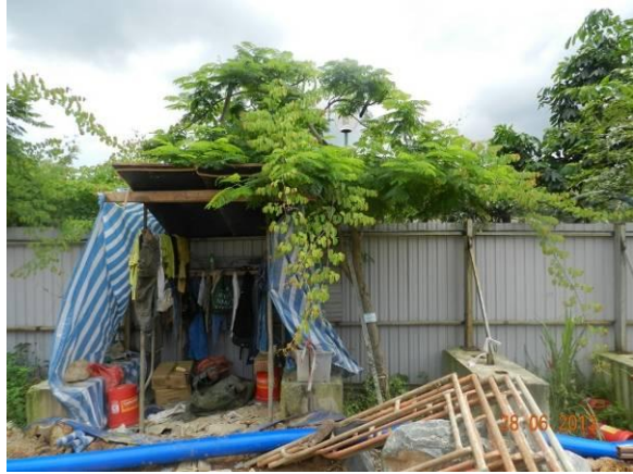
Photo 26 – A temporary shelter has been established next to the relocated tree U74 ( Delonix regia ).
