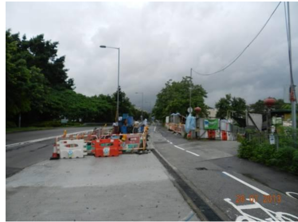
Photo 2 – Temporary barriers established along a section of Ting Kok Road to the south of Area A.
