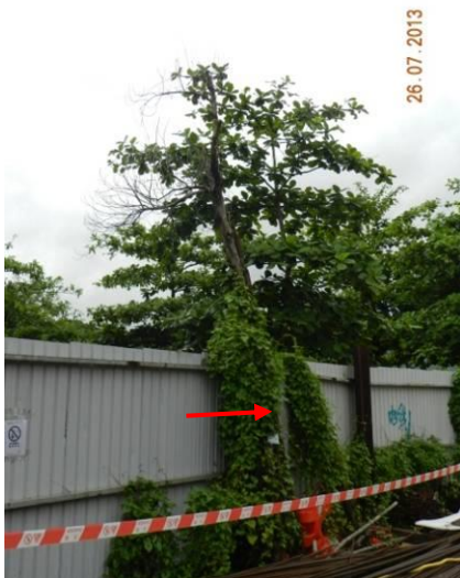
Photo 17 – Very poor condition of the relocated tree T102 as observed within the Phase 2 works area of Area B.
