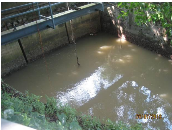
Photo5. Wai Ha River at W2
