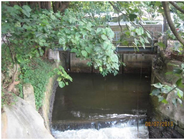
Photo 3. Wai Ha River at W2
