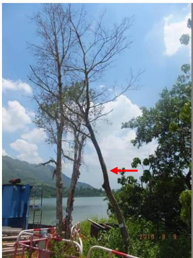
Photo 11 –The relocated E97 was in poor condition as inspected on 9 th August 2013.
