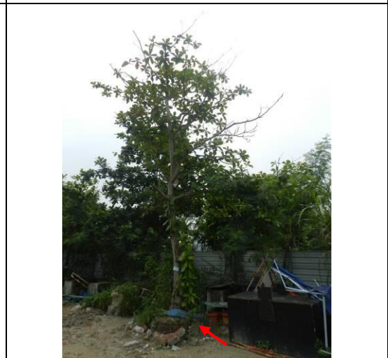
Photo 22 – Half of the planter of U47 was broken.
