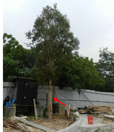
Photo 12 – E38 was recently relocated within Area A and it was guyed by two ropes.
