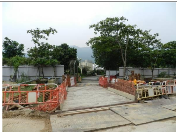
Photo 4 – The temporary hoardings at the eastern end of Phase 1 and the western end of Phase 2 works area were replaced by temporary construction barriers.
