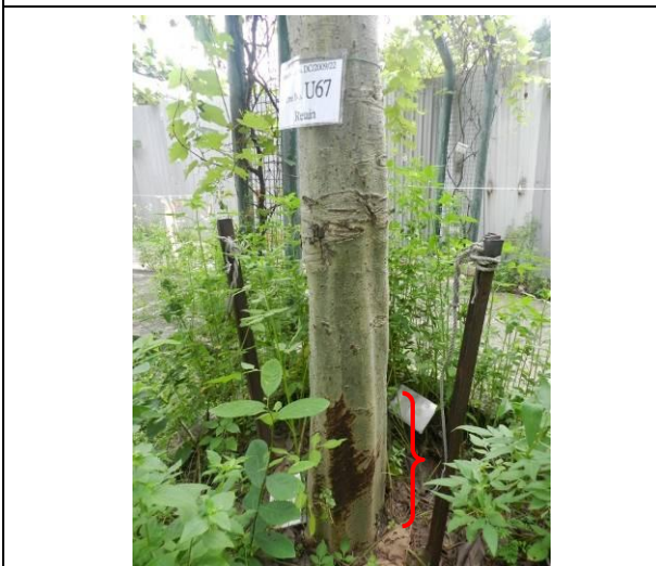
Photo 23 – The retained tree U67 remained in fair condition but sign of suspected termite infestation was noted at its lower trunk.
