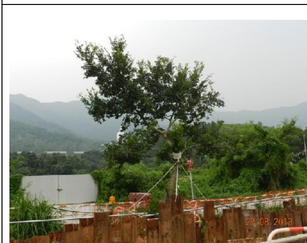
Photo 23 – The retained tree T025 was pruned before and it was temporarily guyed to provide additional support to this tree.
