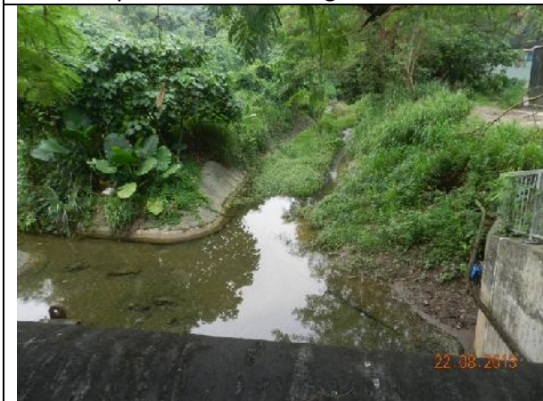
Photo 15 – No direct water discharge into the upper stream of Wai Ha River was observed as the construction works have been concentrated at the lower end of the river.
