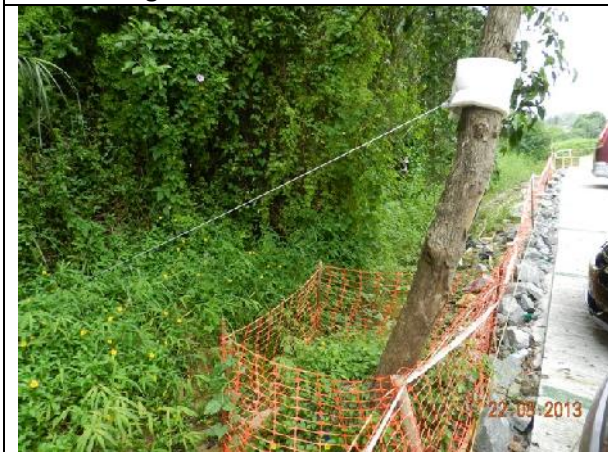
Photo 9 – The untagged leaning tree was guyed at the edge of the parking area within a Tree Protection Zone.
