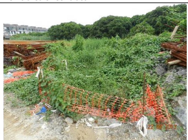
Photo 12 – A sedimentation beds aligned from the area opposite to the Jade View Villa towards the marsh area at southeast. No muddy water was observed but the beds were overgrown by dense grassy vegetation.
