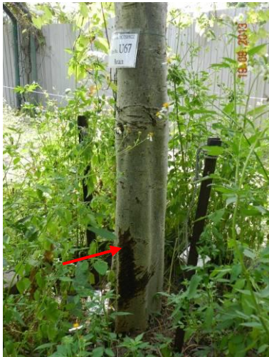
Photo 17 – A sign of suspected termite infestation was observed close to the trunk flare of U67.
