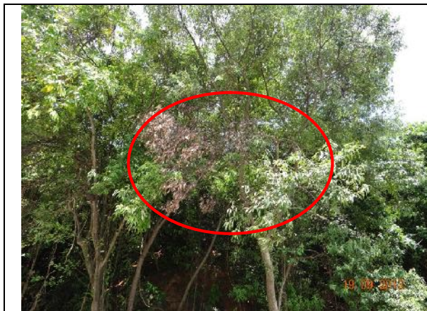
Photo 19 – A broken branch was seen hanging on the retained tree T093.
