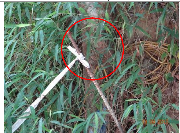
Photo 22 – Tapes and ropes were still found tied on the trunk of the retained tree T103.
