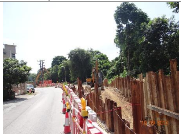
Photo 4 – Sheet piling work in the works area outside the public toilet.
