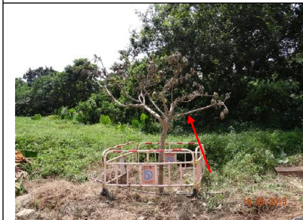
Photo 21 – The retained tree T190 was suspected to be relocated or re-planted and it appeared to be “up-right” but in very poor health condition.
