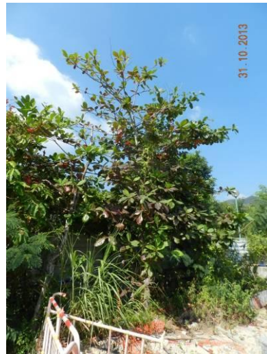
Photo 28 – Overgrown climbers were found on the canopy of U36.
