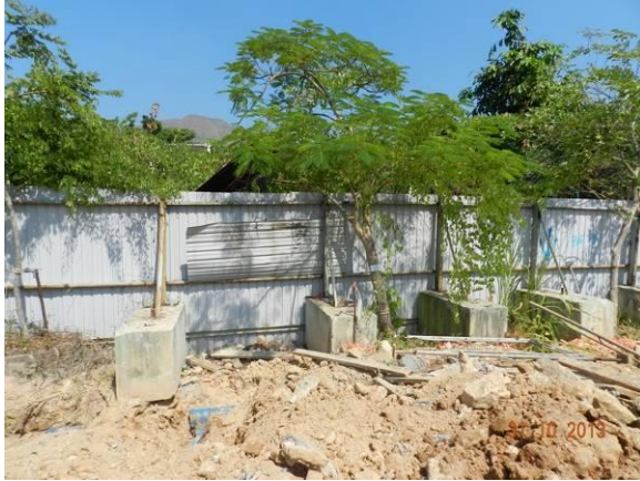
Photo 25 – The temporary shelter next to the relocated tree U74 in Area B was removed.
