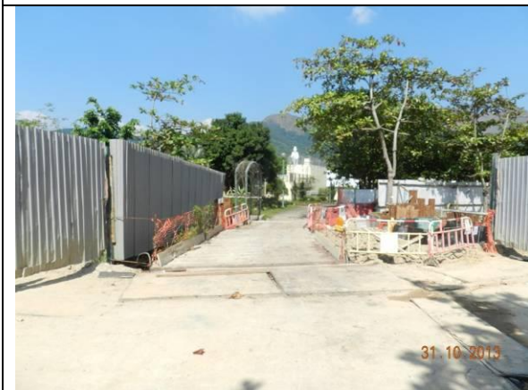
Photo 3 – Temporary construction hoardings had been established along the eastern end of Phase 1 with an entrance and the western end of Phase 2 works area.
