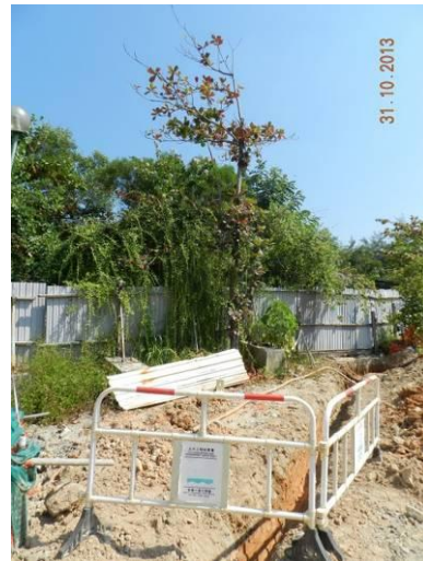
Photo 34 – The excavated work was conducted close to the tree U53.
