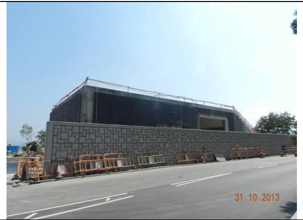
Photo 2 – The permanent boundary wall has been established along the western side of Area A.
