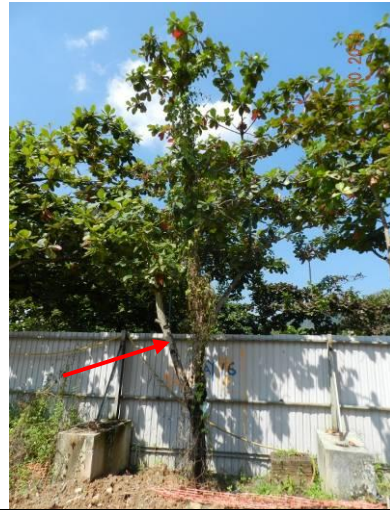
Photo 26 – Dry and cracked tree bark was observed on a topped scaffold limb of U79.
