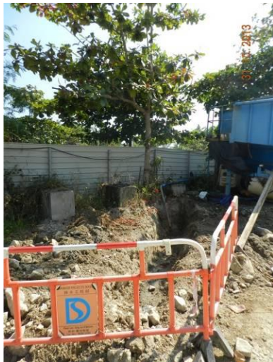
Photo 33 – The excavated work was conducted very close to the tree U54.
