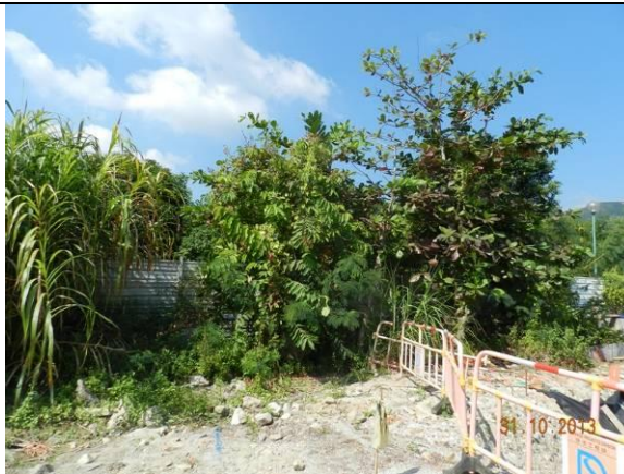
Photo 15 – No more storage of construction material was observed next to the tree groups in Area B.
