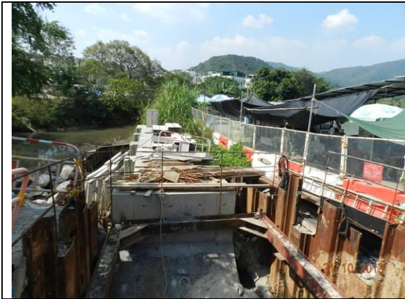
Photo 1 – Temporary hoardings have been established to surround the works area at Wai Ha River estuary.
