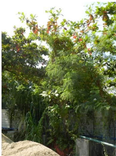
Photo 29 – Overgrown climbers were found on the canopy of U52.
