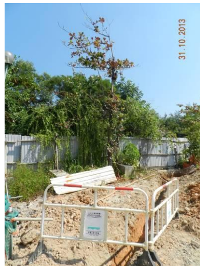
Photo 30 – Overgrown climbers were found on the canopy U53.
