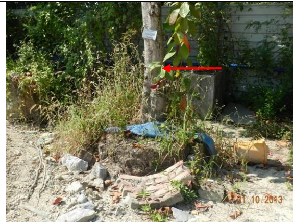
Photo 16 – Half of the planter of U47 was broken and not yet repaired.
