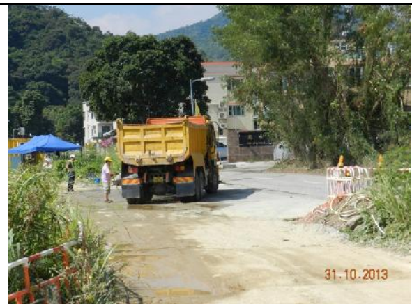
Photo 20 – A new exit for Contract 2 works area was seen opposite to the tree group T021-029 ( Leucaena leucocephala ) and workers were noted washing the wheels of the vehicles which were leaving the works area.
