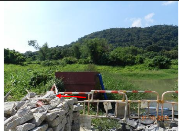
Photo 10 – A filtration tank covered by plastic mat next to the area in October 2013.
