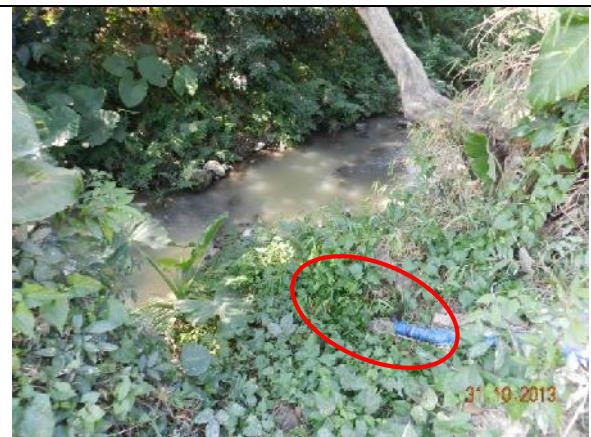
Photo 38 – Some muddy water from the box culvert in the works area was also found pumping to Wai Ha River directly.
