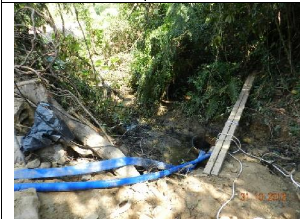
Photo 39 – In the works area at the end of the Treasure Spot Garden II next to the retained tree T103, a stream was blocked and the stream water was pumped to the drainage of the adjacent building.
