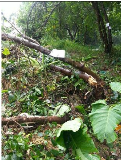
Photo 53 – T184 collapsed and was damaged after the severe typhoon Usagi during 22 nd to 23 rd September 2013. Photo recorded was provided by the Main Contractor.
