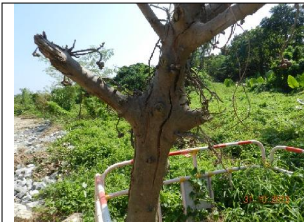
Photo 49 – Loose bark was noted along the trunk and dry fruit was seen on branches of T190.
