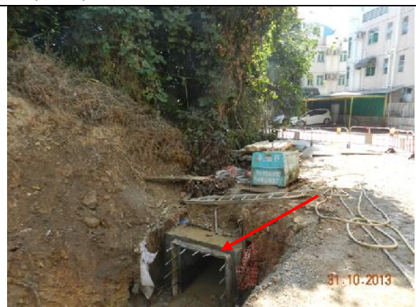
Photo 18 – Excavation work was noted at the end of the Treasure Spot Garden II for joining the old pipe to the new box culvert (Red arrow).
