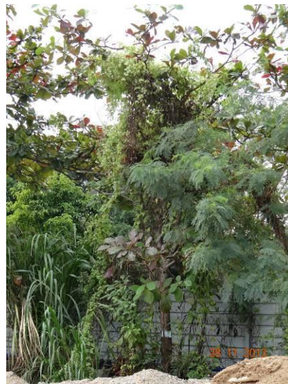
Photo 28 – Overgrown climbers were found on the canopy of U52.
