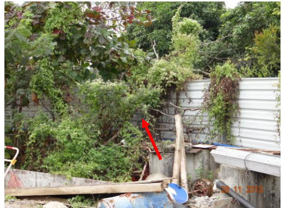
Photo 16 – The dead tree U35 was collapsed in previous month.
