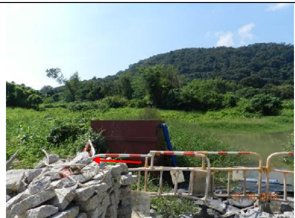
Photo 10 – A filtration tank covered by plastic mat next to the area in October 2013.
