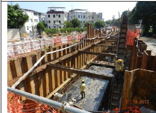
Photo 3 – Construction works for building the box culverts along Tung Tsz Road opposite to Wai Ha outside the public toilet.
