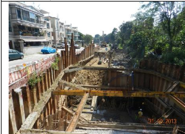
Photo 5 – Construction work was started again along Wai Ha River.
