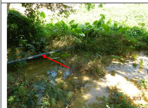
Photo 35 – The pipe was then directed along the river to the grassland behind the tree group T181-183 and the water was then released directly.
