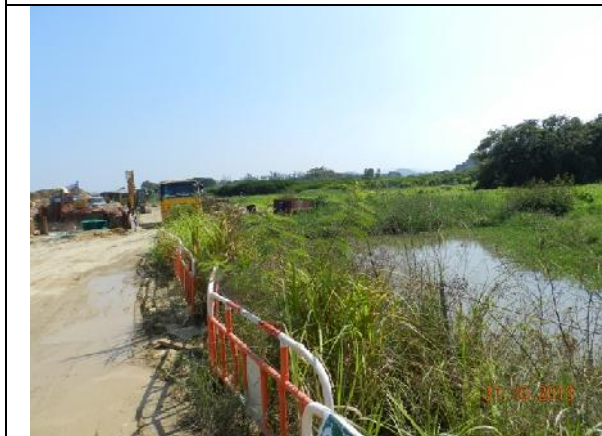
Photo 9 – Temporary construction barriers surrounding the eastern side of the wetland rehabilitation area.
