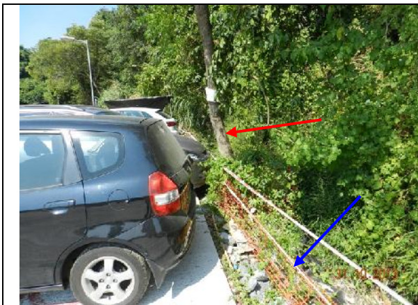
Photo 13 – The untagged leaning tree (Red arrow) was guyed at the edge of the parking area within a Tree Protection Zone demarcated by orange construction nets (Blue arrow).
