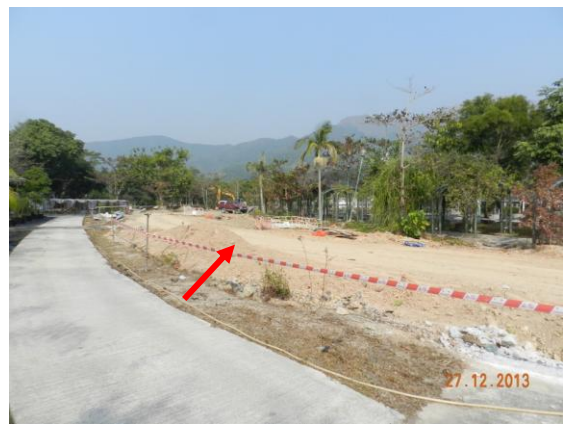
Photo 5 – The temporary construction hoardings in Phase 1 were removed and replaced by barrier tape.
