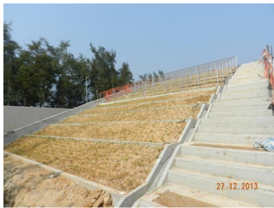
Photo 11 – The slanting component of the pumping house was vegetated with ground cover Arachis duranensis .
