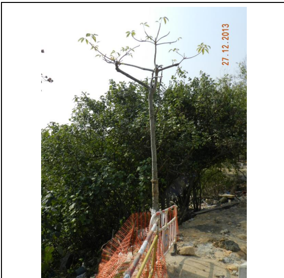
Photo 13 – Tree Protection Zone of E16 was demarcated by construction barriers and nets.
