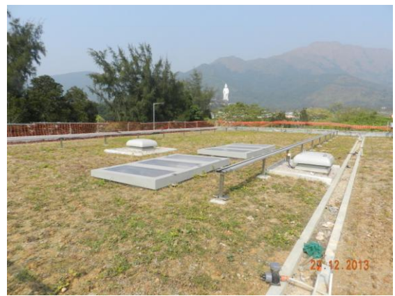
Photo 12 – The rooftop of the pumping house was vegetated with ground cover Arachis duranensis .
