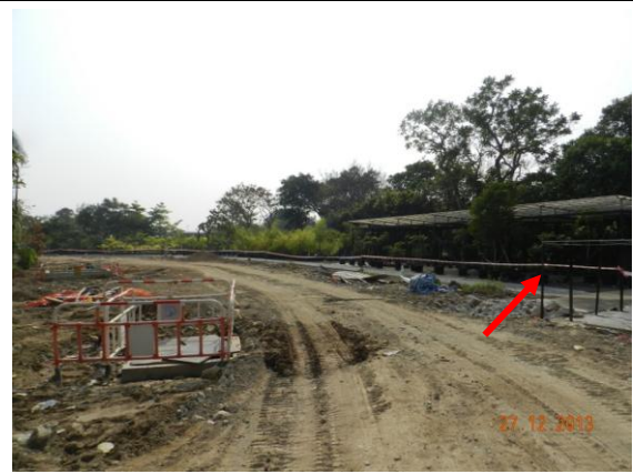
Photo 4 – The temporary construction hoardings in Phase 1 were removed and replaced by barrier tape.
