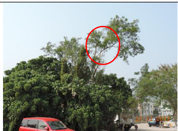
Photo 24 – A broken branch hanging in the canopy of the retained tree T091 was removed.
