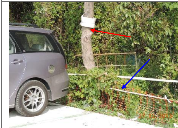
Photo 9 – The untagged tree (Red arrow) was guyed at the edge of the parking area within a Tree Protection Zone demarcated by orange construction nets (Blue arrow).
