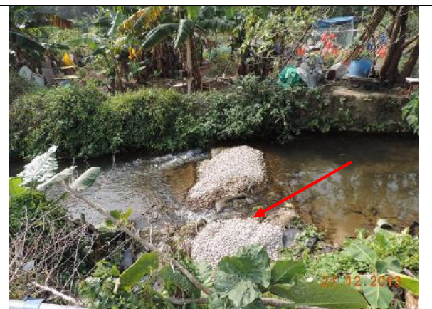
Photo 18 – Sections of granules with underlaid PVC liners were found along the river for further sedimentation but several sections of granules were washed away.
