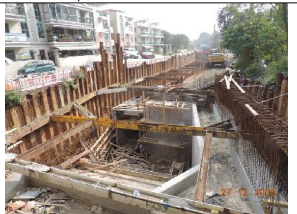
Photo 4 – Construction work continued along Wai Ha River.
