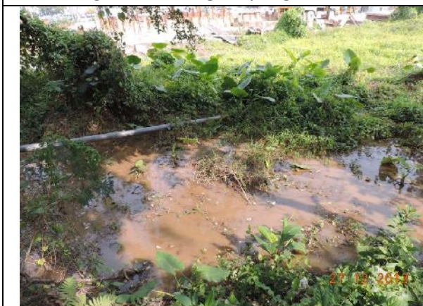
Photo 17 – The water from the sedimentation tank was directed along the river to the grassland behind the tree group T181-183. The discharge was clear in December 2013.
