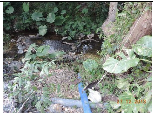
Photo 20 – Water from the box culvert in the works area outside the public toilet was noted pumping out and releasing to Wai Ha River.
