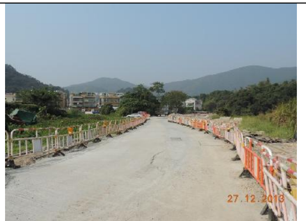
Photo 2 – Temporary hoardings have been erected along the access road from Tung Tsz Road to Treasure Spot Garden II.
