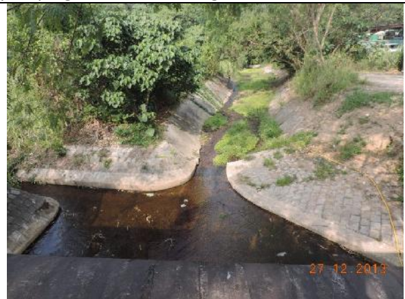
Photo 22 – No direct water discharge into the upper stream of Wai Ha River was observed as the construction works have been concentrated at the lower end of the river.
