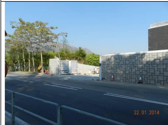
Photo 3 – Construction of the proposed boundary walls along part of the northern and western sides of Area A was in progress.
