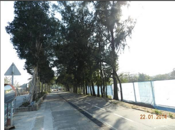
Photo 8 – Chain-link fence was reinstated at the eastern end of Phase 2 work area and covered by canvas sheets.
