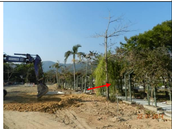
Photo 34 – The trunk of the transplanted tree U53 was tied tightly by strings and a hessian wrapping which was left after the transplantation of the tree.
