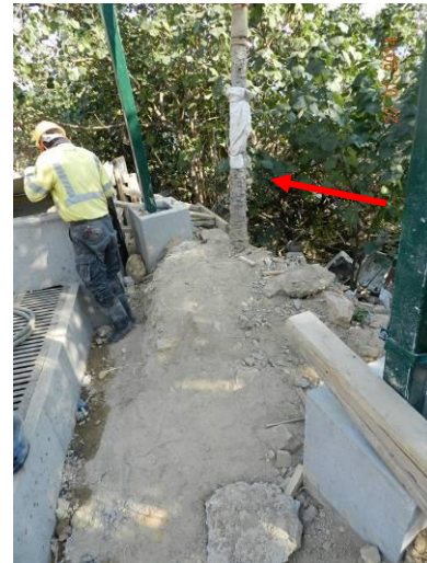
Photo 16 – Soil grade change was observed around the trunk base of E16 and minor exposed roots were found.
