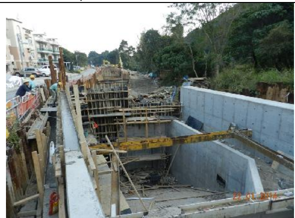
Photo 4 – Construction works continued along Wai Ha River.
