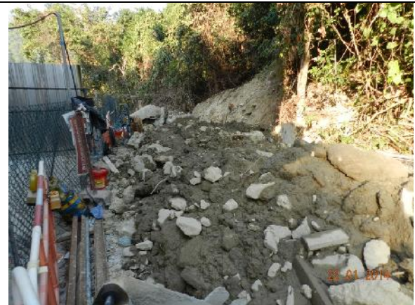
Photo 10 – Works were observed at the end of the Treasure Spot Garden II near the retained tree T103 and the works area was surrounded by temporary construction barriers and chain-link fence.
