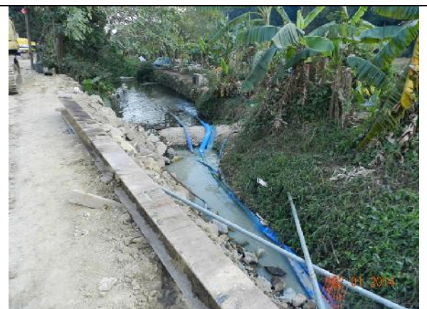
Photo 18 – The discharge from the sedimentation tank was released back to the sections of granules with underlaid PVC liners along the river. The discharge was seen unclear when released and then became clean after filtration.
