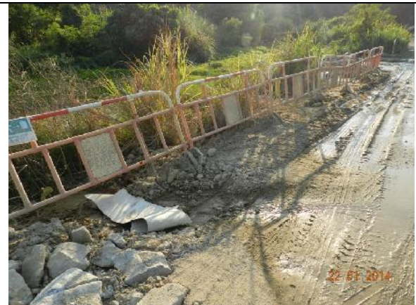
Photo 6 – Temporary construction barriers surrounded the eastern side of the wetland rehabilitation area.
