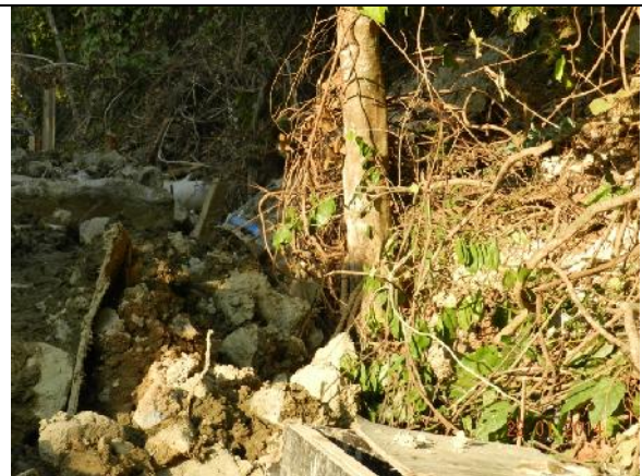
Photo 28 – Excavated soil and rocks were noted piling close to the trunk base of the retained tree T103.
