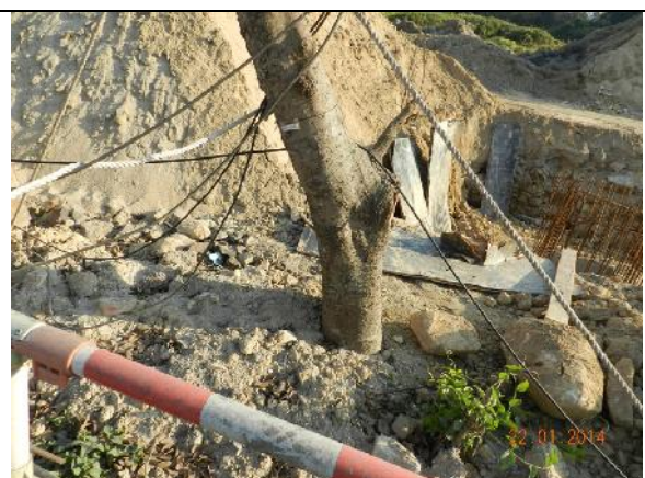
Photo 30 – Excessive soil was still piled around the root flare of T025.
