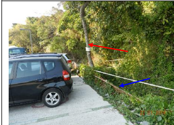
Photo 9 – The untagged tree (Red arrow) was guyed at the edge of the parking area within a Tree Protection Zone demarcated by orange construction nets (Blue arrow).
