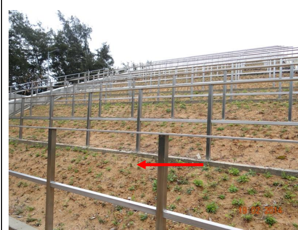
Photo 15 – The proposed green roof of the pumping house was vegetated with ground cover Arachis duranensis .
