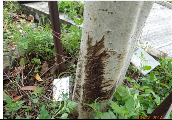
Photo 32 – Sign of suspected termite infestation was observed at the lower trunk of U67.
