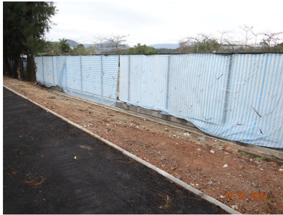
Photo 9 – Chain-link fence was reinstated at the eastern end of Phase 2 works area and covered by canvas sheets.
