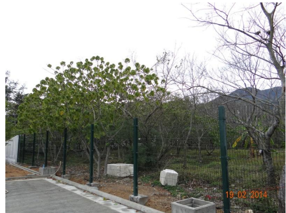
Photo 4 – Proposed chain-link fence has been erected along the rest of the boundary sides of Area A.
