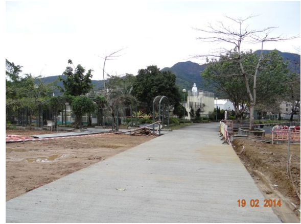
Photo 8 – The open section between Phases 1 and 2 works areas was opened again after the reinstatement works.
