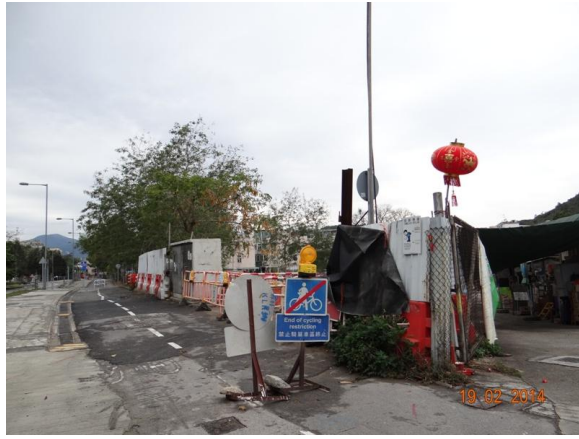
Photo 1 – Temporary construction hoardings have been established around the works area at Wai Ha River estuary.
