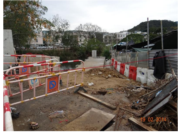
Photo 2 – Temporary construction hoardings have been established around the works area at Wai Ha River estuary.
