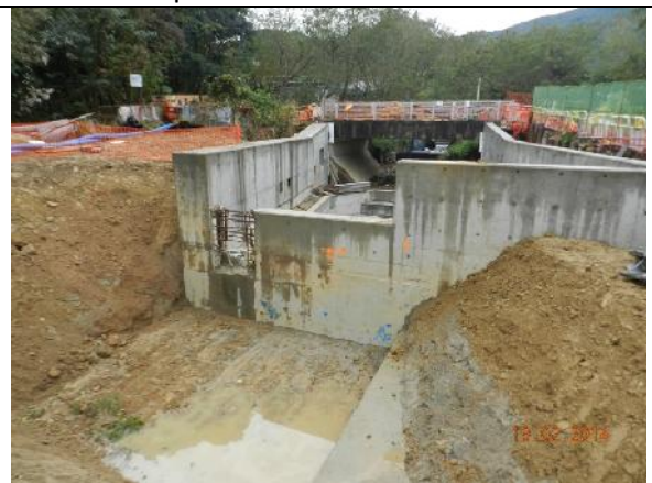
Photo 4 – Construction works continued along Wai Ha River.
