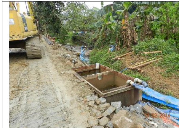
Photo 15 – No more muddy water from the works area was pumped to the sedimentation tank settled at the end of the works area.
