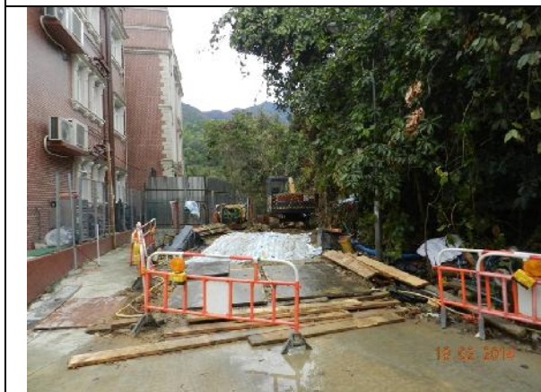
Photo 9 – Works were observed at the end of the Treasure Spot Garden II near the retained tree T103 and the works area was surrounded by temporary construction barriers and chain-link fence.
