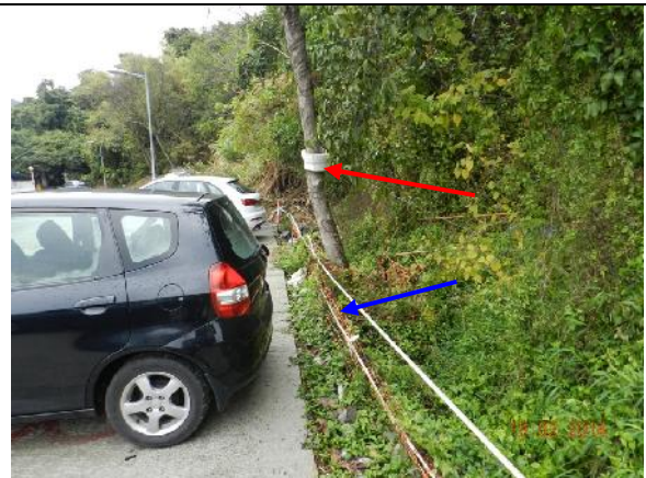
Photo 8 – The untagged tree (Red arrow) was guyed at the edge of the parking area within a Tree Protection Zone demarcated by orange construction nets (Blue arrow).
