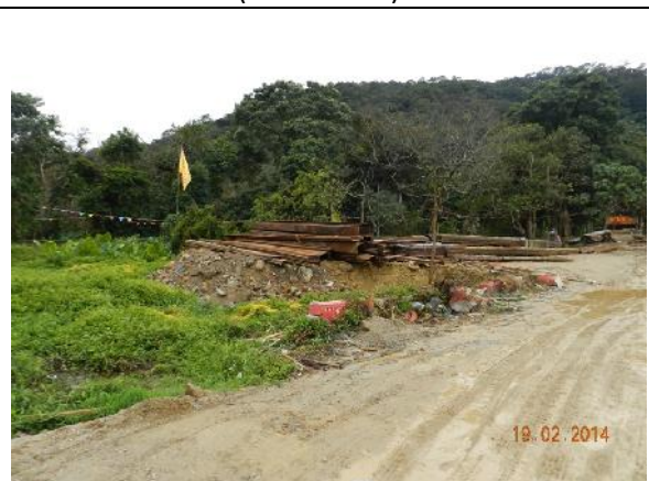
Photo 10 – The expanded works area near the previous collapsed tree T190 ( Ficus hispida ) was still used for storage of construction materials.
