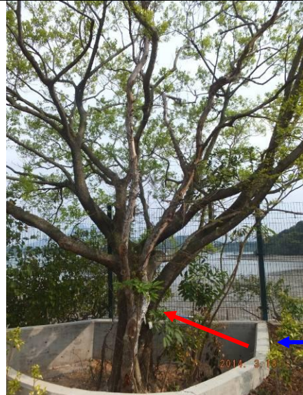
Photo 20 – The retained tree T253 was in poor condition (red arrow). A planter (blue arrow) was built to protect the retained trees T253 and E63.
