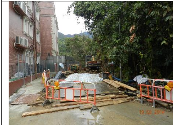
Photo 9 – Works were observed at the end of the Treasure Spot Garden II near the retained tree T103 and the works area was surrounded by temporary construction barriers and chain-link fence.
