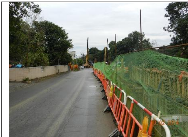
Photo 1 – Temporary hoardings have been erected along Tung Tsz Road opposite to Wai Ha.
