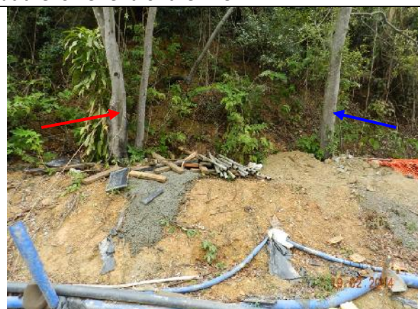
Photo 24 –Storage of construction materials was noted close to the trunk flares and trunks of T093 (Red arrow) and sand piling was seen close to the trunk flare of T094 (Blue arrow).
