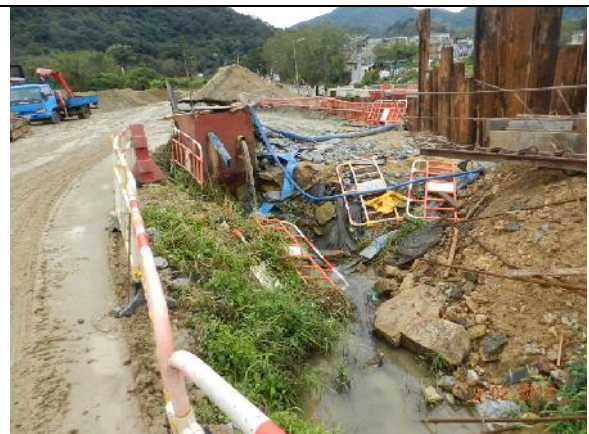
Photo 12 – A sedimentation tank was seen receiving the waste water from the works area near the previous collapsed tree T196 and the discharge was seen to be clear.
