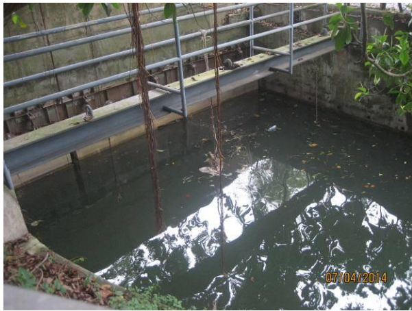
Photo 3. Wai Ha River at W2
