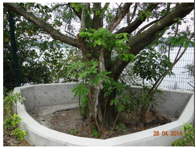
Photo 16 – Example of built planting area to protect the retained trees (T263 and E63).
