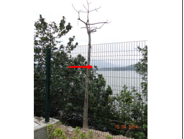
Photo 18 – The relocated E16 was in marginally fair condition and separated outside the chain-link fence.
