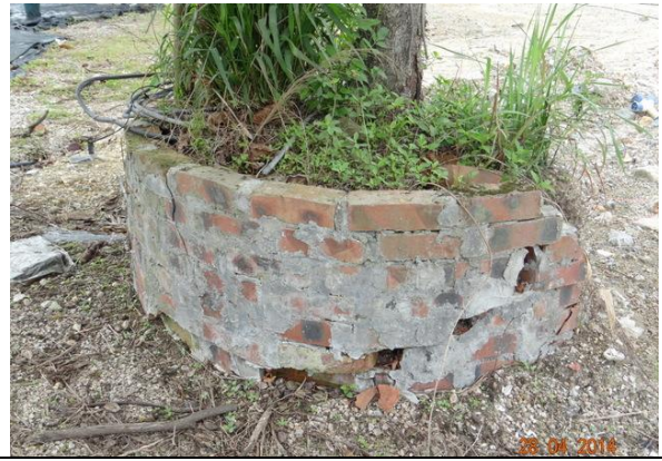
Photo 26 – The planter of another untagged Terminalia catappa next to U54 was broken, with exposed roots and soil.
