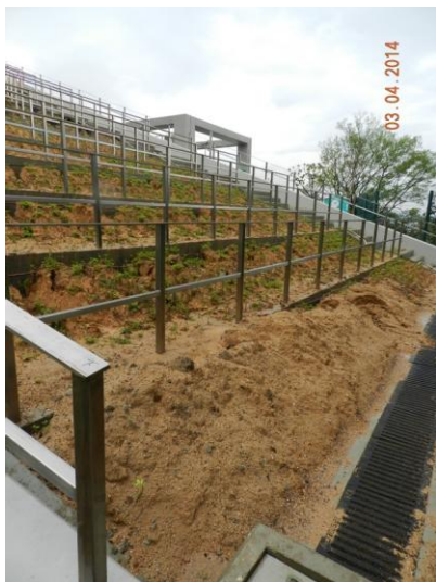
Photo 11 – The soil was washed away from the planting area down to the bottom of the pumping house as observed on 3 rd April 2014.
