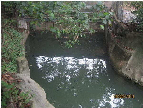
Photo 5. Wai Ha River at W2
