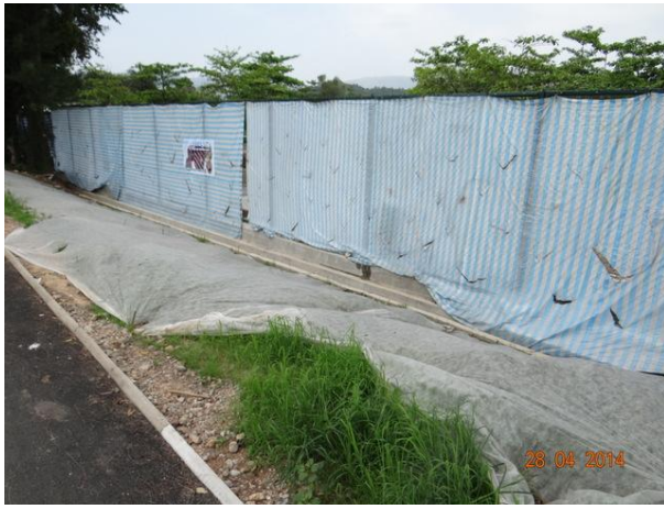
Photo 7 – Chain-link fence was reinstated at the eastern end of Phase 2 works area and covered by canvas sheets. Grass germination was noted in the hydroseeded area applied next to the fence.
