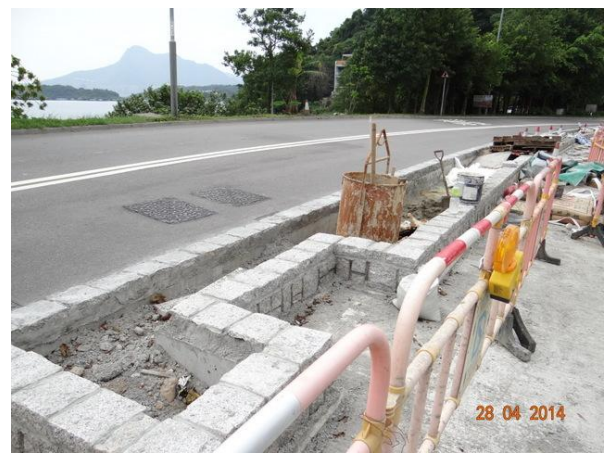
Photo 4 – Construction of a roadside planter along Ting Kok Road.
