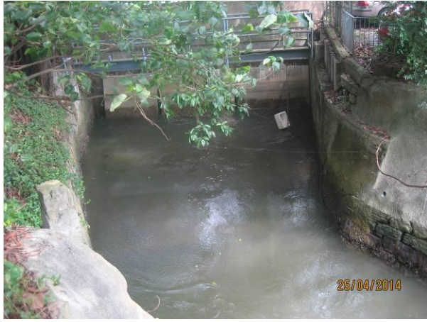
Photo 7. Wai Ha River at W2
