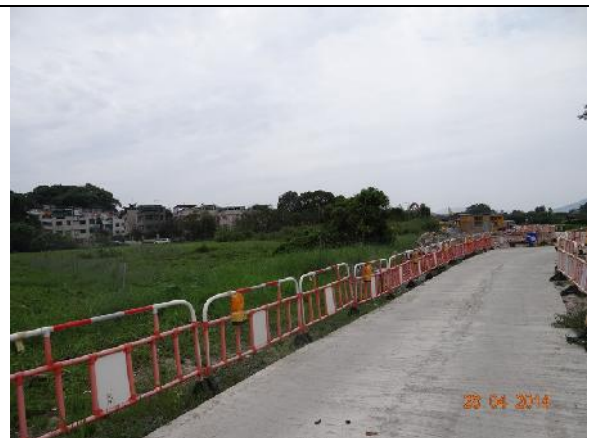
Photo 2 – Temporary hoardings have been erected along the access road from Tung Tsz Road to Treasure Spot Garden II.
