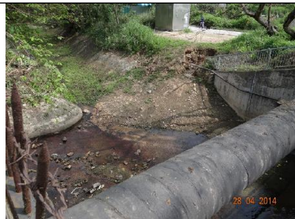
Photo 20 – No direct water discharge into the upper stream of Wai Ha River was observed as the construction works have been concentrated at the lower end of the river.
