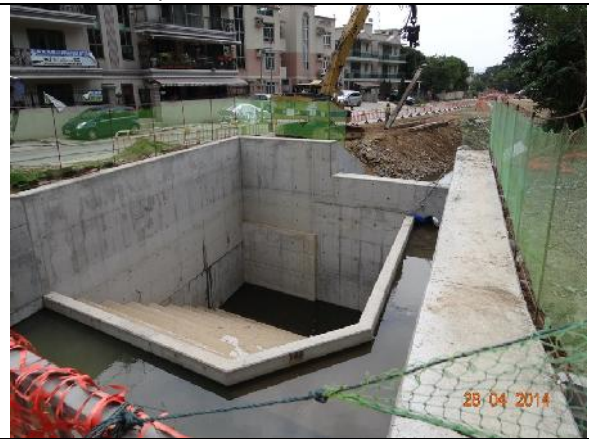
Photo 4 – Construction works continued next to Wai Ha River.
