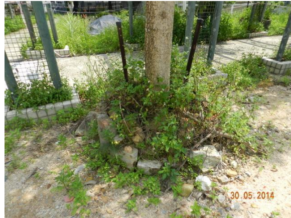
Photo 26 – Close-up view of the broken planter of U69.
