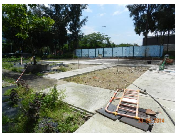
Photo 6 – Phase 1 area of Area B was demarcated by loosened barrier tape, and no reinstatement work was in progress as observed in May 2014.
