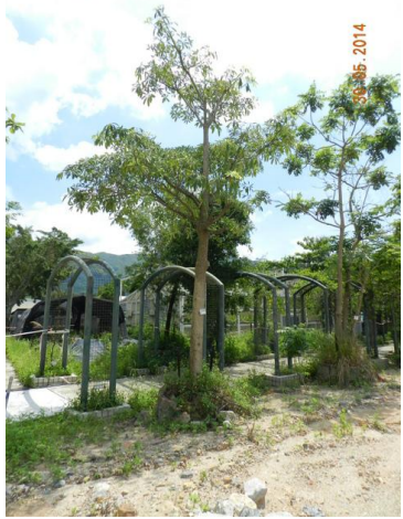
Photo 25 – The planter of U69 ( Alstonia scholaris ) was broken and the exposed roots and soil were observed.
