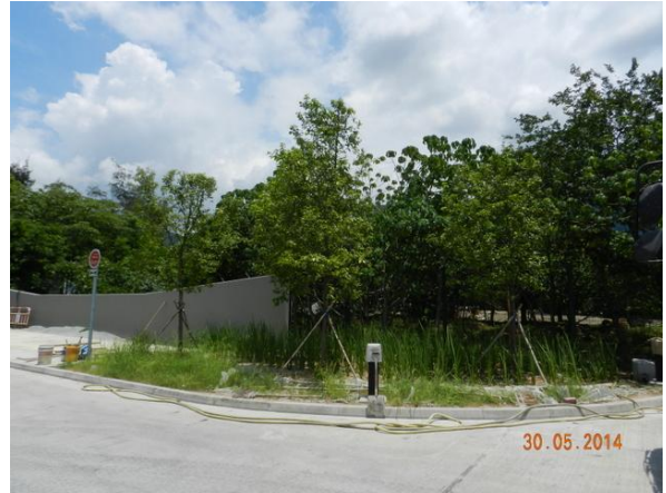
Photo 14 – The planted trees Cinnamomum burmannii and ground cover Iris tectorum were in fair condition.
