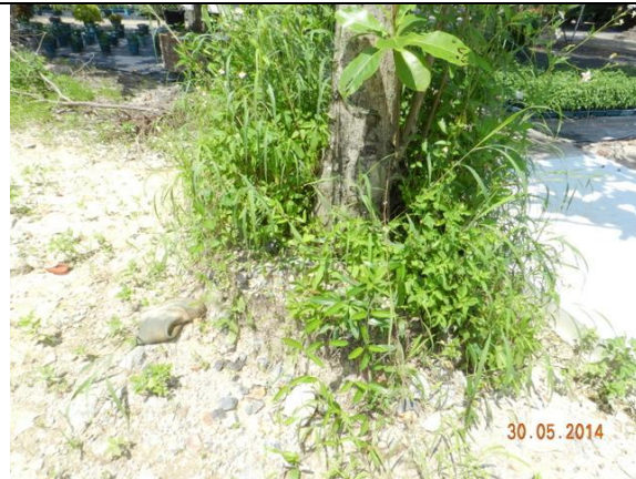
Photo 21 – Close-up view of the broken planter of U47.
