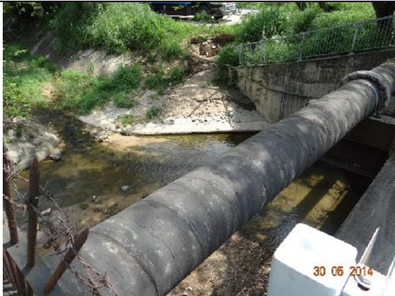
Photo 17 – No direct water discharge into the upper stream of Wai Ha River was observed as the construction works have been concentrated at the lower end of the river.
