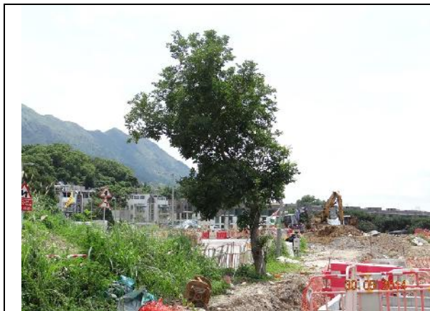
Photo 25 – The retained tree T025 was temporarily guyed to provide additional support to this tree.
