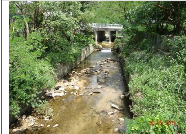
Photo 5 – The sand bags used to divide the river were removed.
