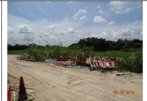
Photo 6 – Temporary construction barriers surrounded the eastern side of the wetland rehabilitation area.
