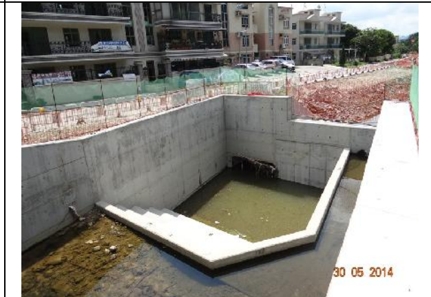
Photo 4 – Construction works continued next to Wai Ha River.
