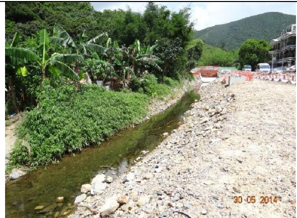
Photo 14 – The river water was noted clear near the tree group T119-122.
