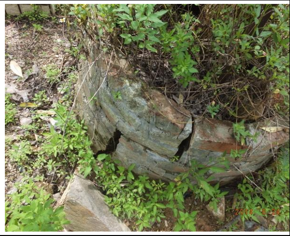
Photo 26 – Close-up view of the broken planter of U69.
