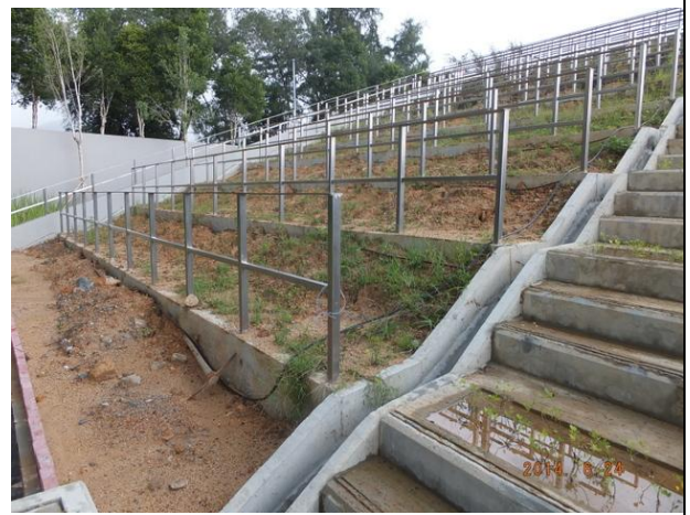
Photo 10 – The growth of the ground cover planted on the slanting component of the green roof was generally slower.
