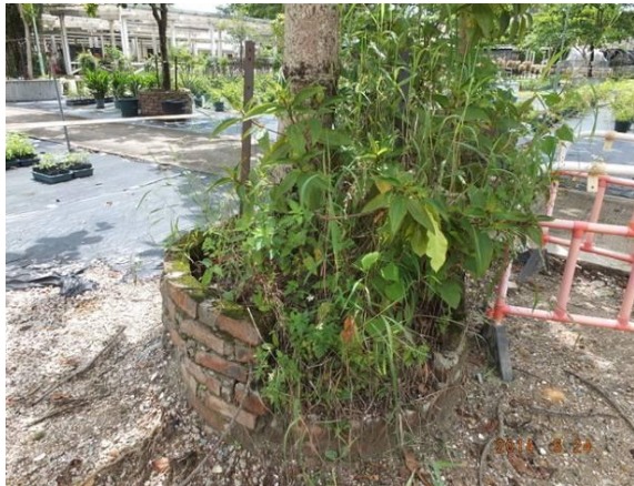
Photo 23 – The planter of U54 ( Terminalia catappa ) was broken and the exposed roots and soil was observed.
