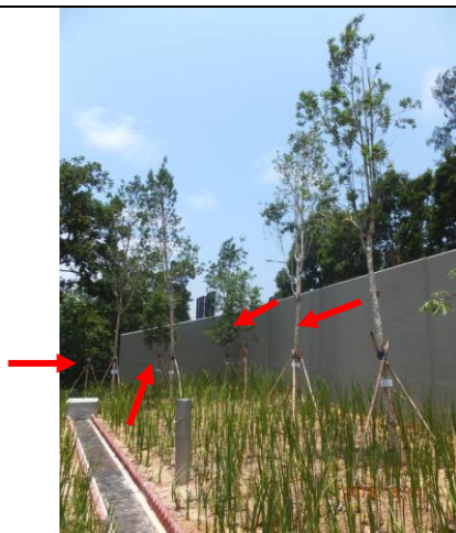
Photo 17 – The four newly replaced trees Melaleuca cajuputi subsp. cumingiana at the southeastern corner were in fair condition.
