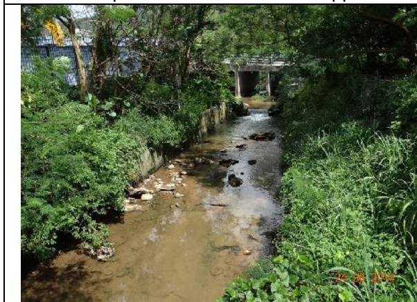
Photo 5 – The sand bags used to divide the river were removed.
