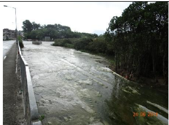
Photo 18 – The area opposite to Jade View Villa to the exit point near Shuen Wan Tung Tsz Children's Playground was covered by a mat. The area was waterlogged and unclear water overflowed into the nearby marsh area.
