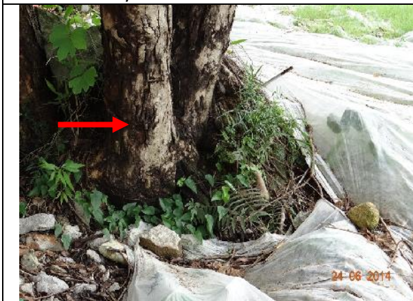
Photo 29 – Excavation work was noted next to an untagged tree ( Cleistanthus nervosum ) (Red arrow). Severe exposed roots were noted on this tree.
