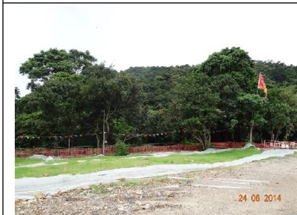
Photo 11 –The construction materials stored on the works area near the location of the previously removed tree T190 ( Ficus hispida ) were removed. This area has been covered by a mat in May 2014 and hydroseeding was applied in June 2014.
