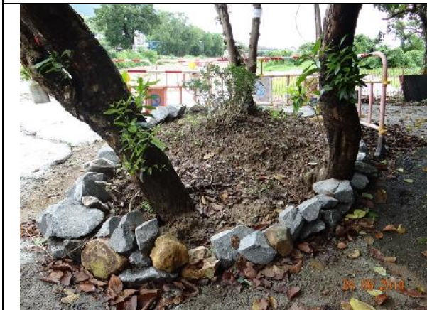
Photo 27 – Excavation work was noted very close to the tree group T181-T183. Excavated soil was noted piling around their trunk flares and the orange construction nets covered on the three trees were removed. These trees have been surrounded by some stones.
