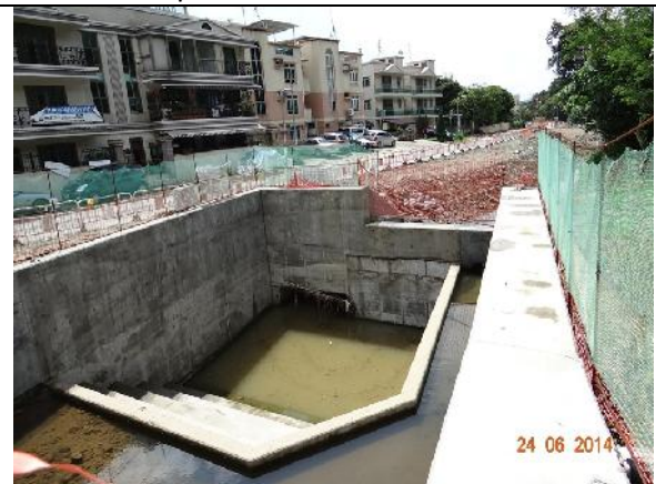
Photo 4 – Construction works have been stopped next to Wai Ha River.
